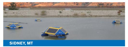
Sidney, MT has four Deep-Flo units in a three acre by 15' deep pond with 5-7 days retention. Waste is 30-50,000 mg/l of BOD from sugarbeet processing waste. This lagoon is in essence an anaerobic digester without a cover. Sunflo2 units have documented uniform temperatures top to bottom (no stratification). A Sunflo2 Floating Sensor Platform Model was recently added to document pH and ORP values to provide the operator information on an hourly basis for flow or chemical adjustment.
