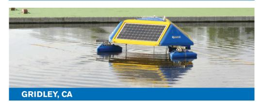
Installed to reduce and redistribute sludge in the effluent and increase dissolved oxygen in waste being transferred from turbulent aeration in the primary pond. Initial response has been favorable, documenting an increase in dissolved oxygen from 0.2 ppm to 1.5-2.0 ppm in first 48 hours.
