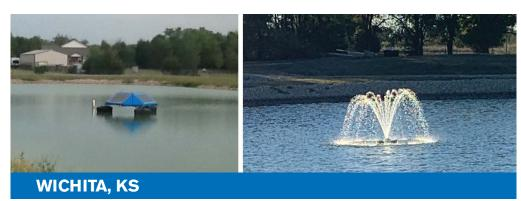
Two fountains placed in adjoining ponds, powered by one solar powered unit. Fountains have increased evaporation and appearance to minimize complaints by nearby home-owners and reduce the need to discharge.
